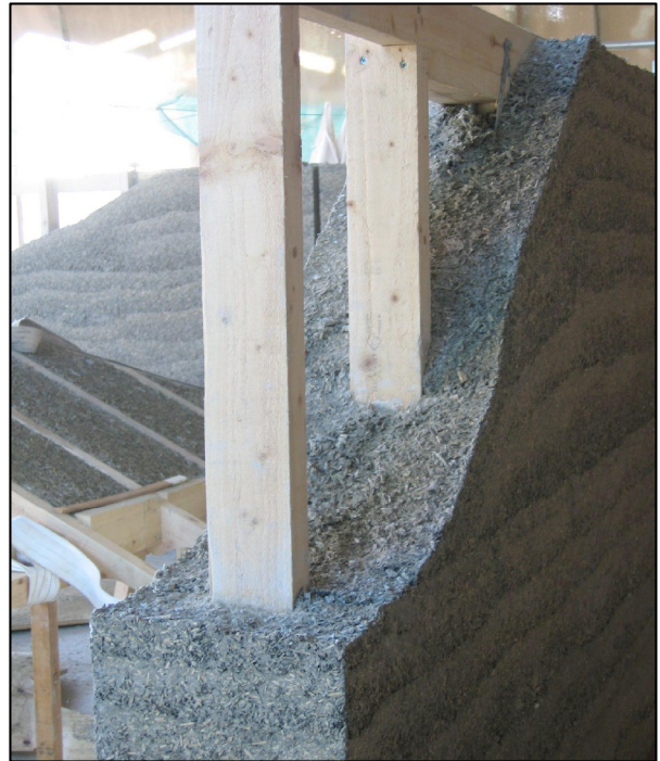
Figure 2.7 - Lime-hemp on a timber frame
