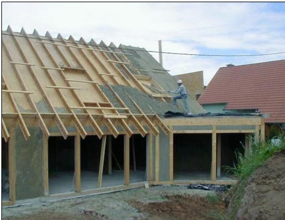
Figure 2.8 – Lime-hemp as roof insulation
